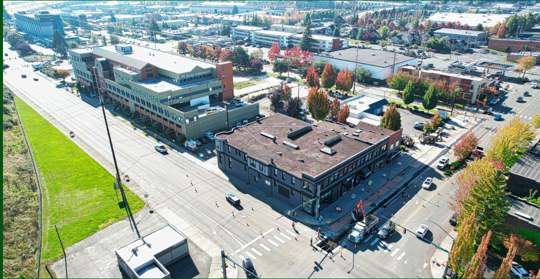
VIEW LOOKING I-5 WEST
