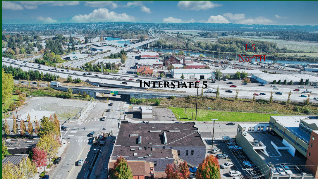
VIEW LOOKING I-5 EAST
